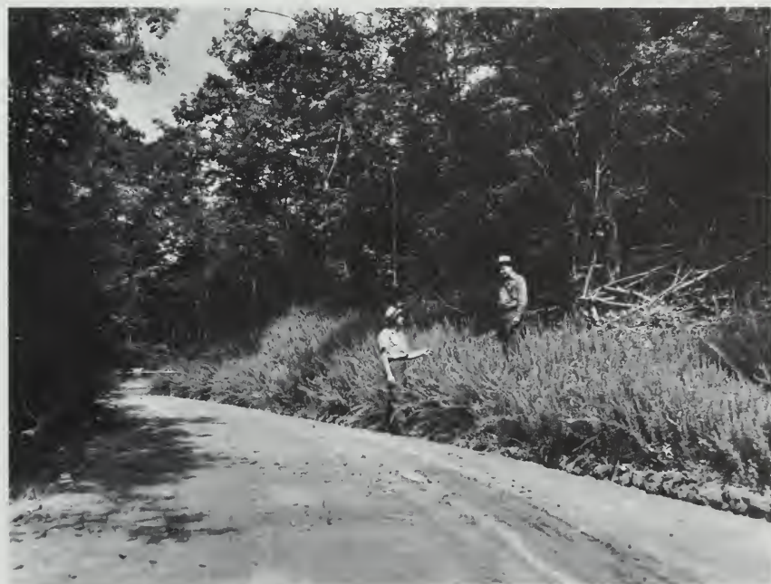
Mr. Seely and Dixie Howell, assistant supervisor of the North Carolina National Forests, inspect plantings that stabilize roadbanks.
